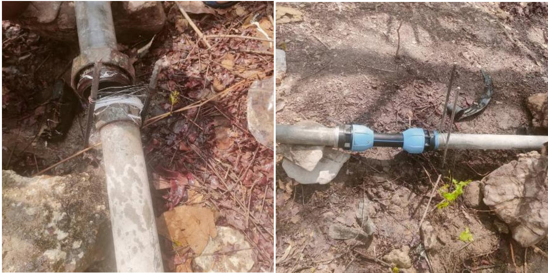
Failed barrel union. All old union components removed, pipe threads repaired, new fittings and pipe installed.
