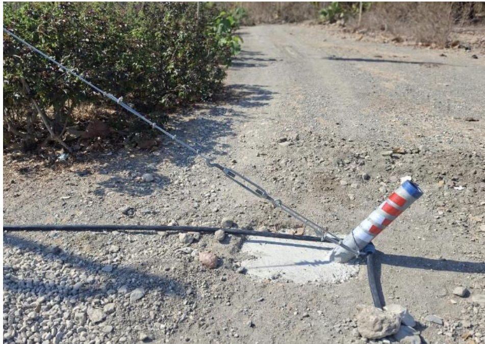
The western bank anchorage.
