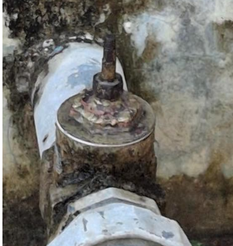
Welded tap-head installed – no leaks!
