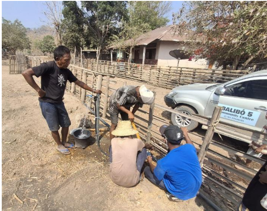
First tap installed in the village. We had not even finished installing it, and it was already being used. Happy villagers! Mario showing the workers how to install the fittings.
