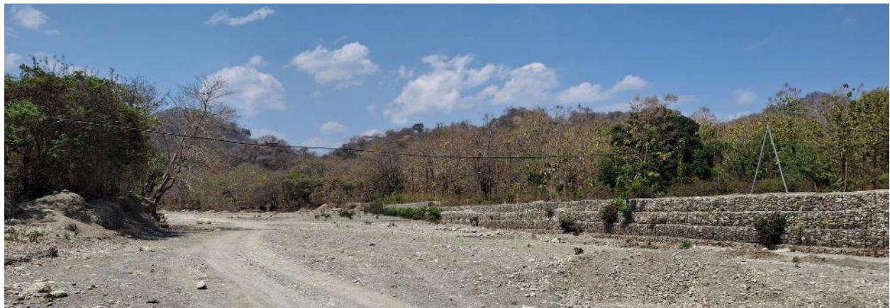
The ropeway erected, with poly pipe attached below it. 5m (+) above river bed.
