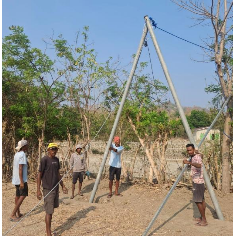
Support structure on the eastern bank raised and inserted into holes ready for concreting. (Legs are 100mm diameter x 6m long steel pipes.) Steel wire rope ready-run through top pulley.
