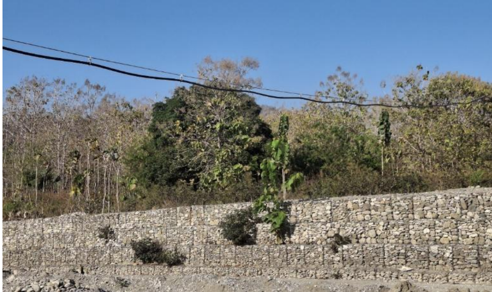
The poly pipe suspended below the steel wire rope.
