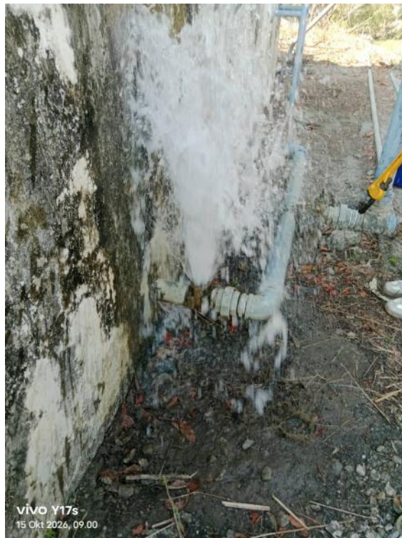
Attempting to install the welded tap-head. Water shooting out of the gate valve – proof the big tank was filling.
