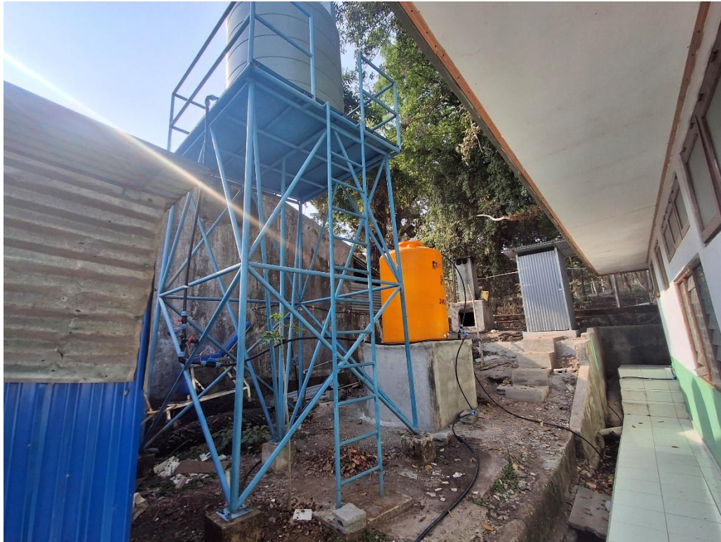
Completed work. Green holding tank ("dirty" water), with water flowing through SkyHydrant in shelter shed, and then to the yellow ("clean" water) tank, which is in turn connected to the Maternity Ward.
