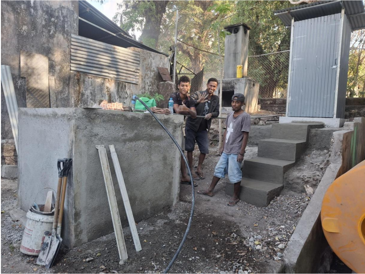
Tank stand rendered; shelter house, slab and steps constructed.
