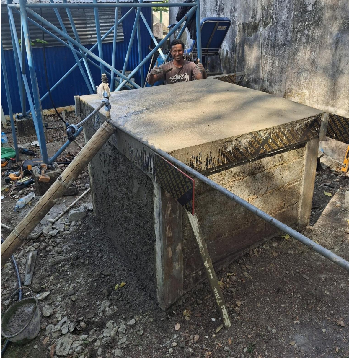
Old tank removed; sides bricked up; and new slab laid on top
