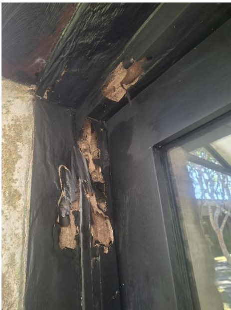
Severe white ant damage in door frames at the Museum
