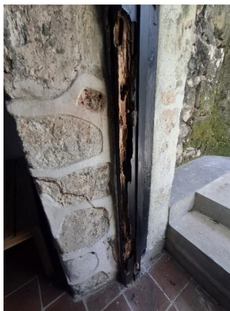
Severe white ant damage in door frames at the Museum
