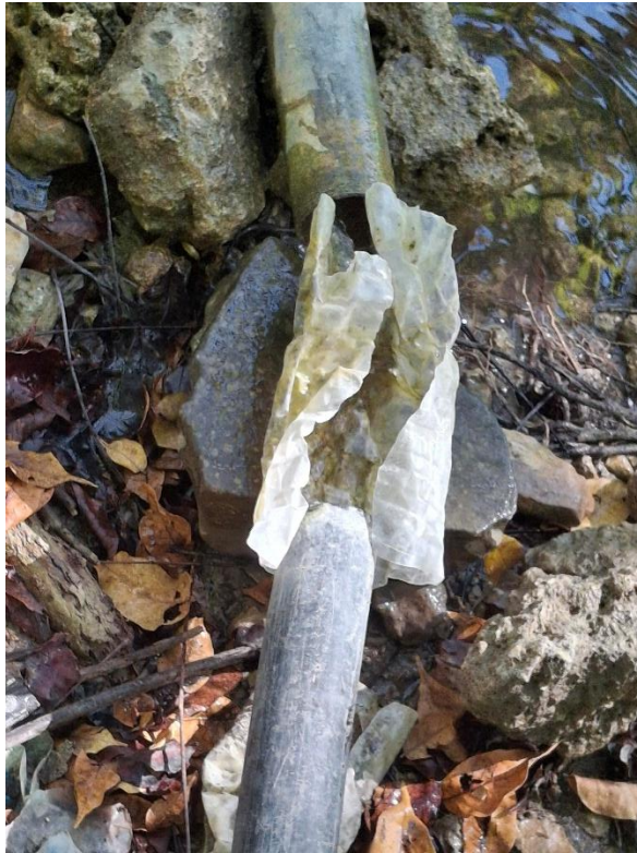
Plastic water bottle transferring water between pipe sections
