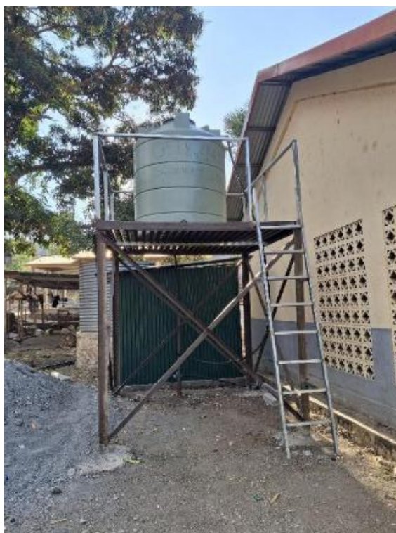
The “dirty water tank” installed on the tank stand, with ladder and safety rails. In the green shed is the pump and SkyHydrant filter system.
