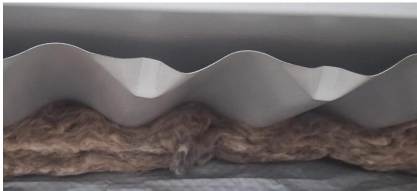
Photo showing the ends of roofing sheets that have been “turned up”.
