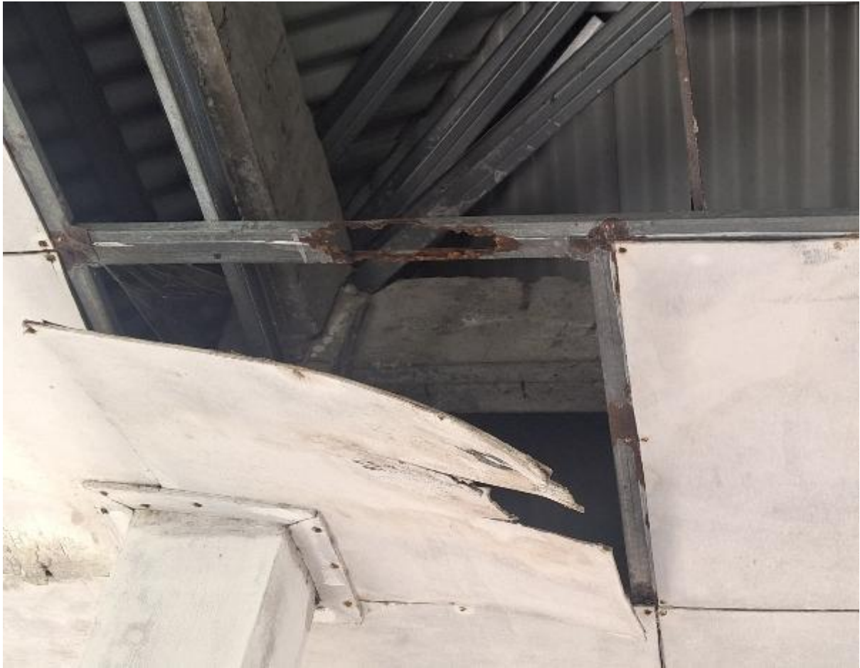
Ceiling batten (to which ceiling sheets are screwed) almost completely rusted away. Note that the actual roof sheeting (not the ceiling sheeting) looks in good condition.
