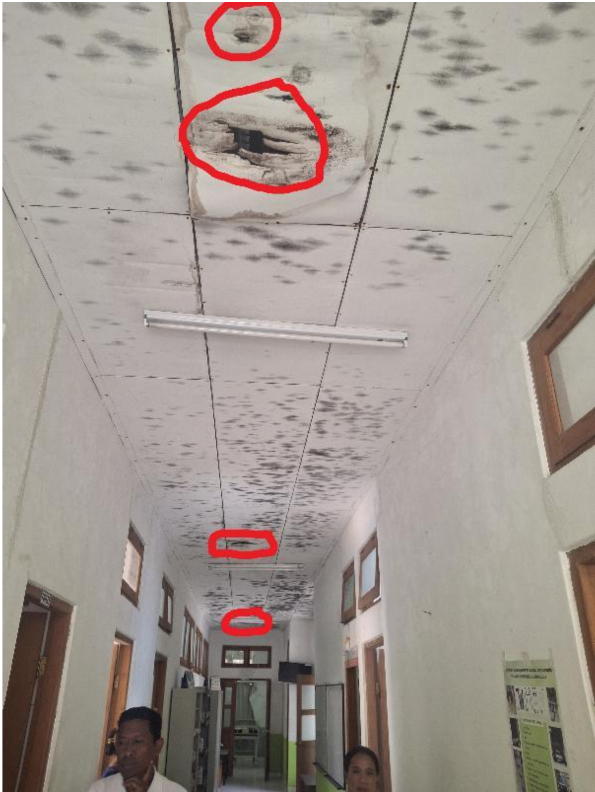
Photo along the central hallway showing the black mould and several areas of water damage (indicated by the red circles). The water damage along the hallway indicates that water is entering via the central part of the roof line – ie the ridge capping area.
