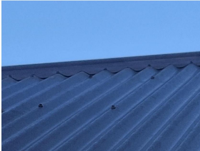
Photo of how the ridge capping should be finished, with the notching completed.
