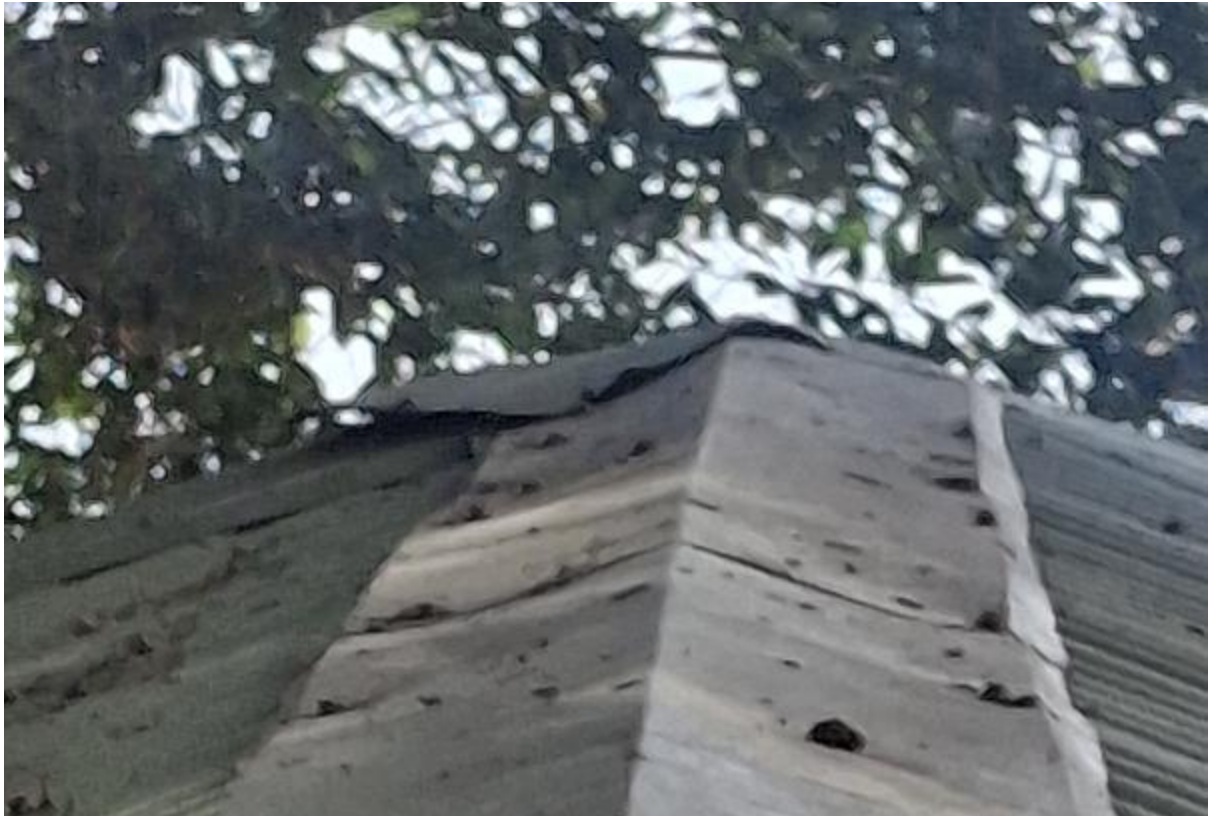
Photo showing ridge capping not secured down.
