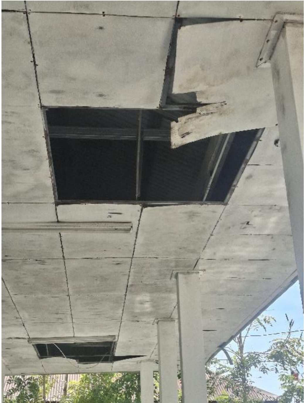
External ceilings badly water damaged, with the damage below the sloping ridge lines.
