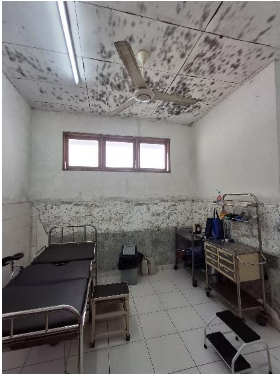
One of the birthing rooms. Most tiles have fallen off the walls (some tiles remaining in the left corner). "New" birthing bed!
