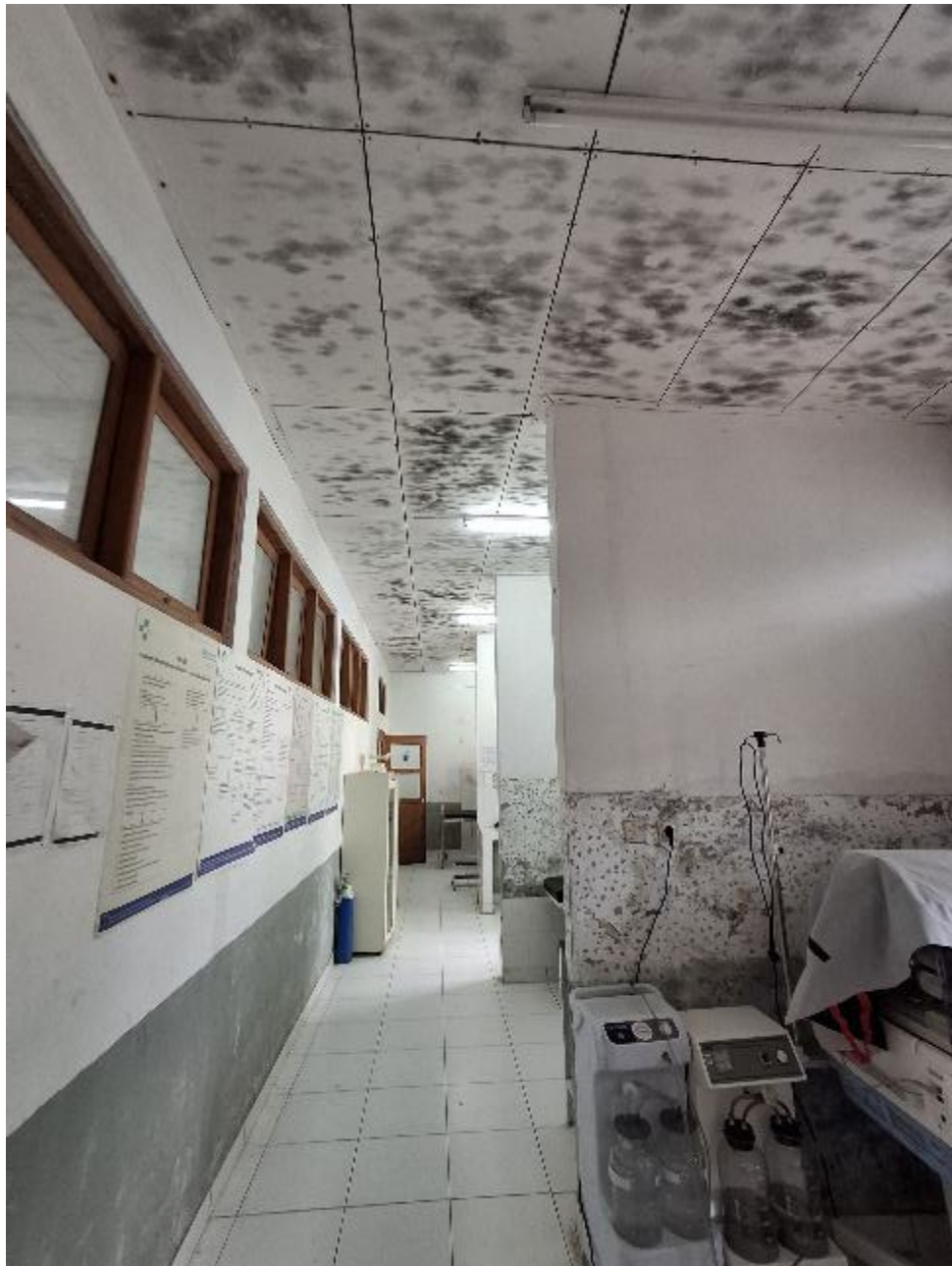
Black mould through the actual birthing rooms. Tiles fallen off the lower parts of the walls.
