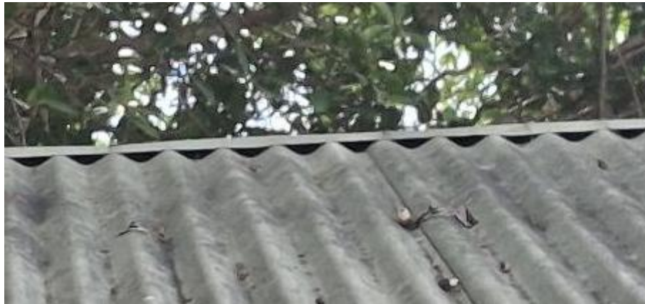
Photo of existing ridge capping
