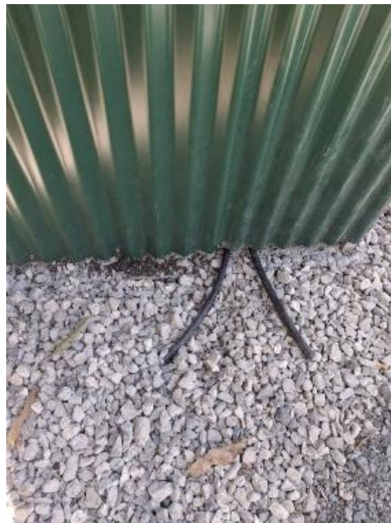
Absorption pit filled with gravel outside shelter house – to take backwash and over-filling water.
