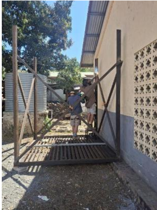
Legs and bracing being added
