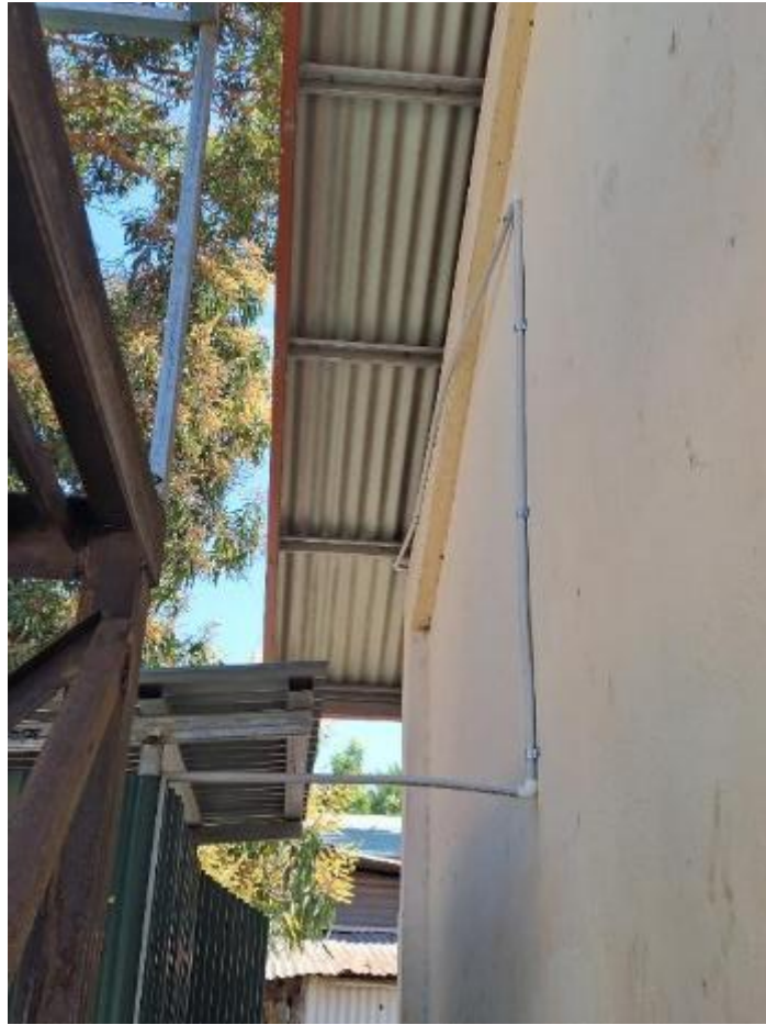
Power cable encased in conduit coming into shelter house.
