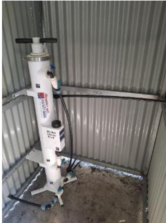
The SkyHydrant Ultra-filtration unit plumbed in and bolted to shelter house wall
