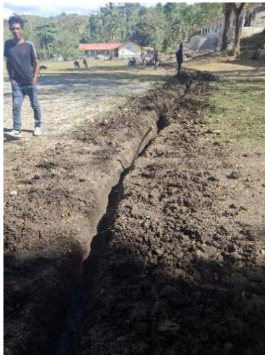
The 300mm deep trench into which the 600m of 50mm poly pipe supply line will be laid.
