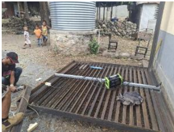
Top platform of tank stand being fabricated (upside down).
