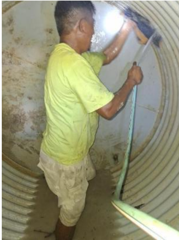
Local neighbour INSIDE the existing clean water tank – washing it and removing about 25mm depth of sandy silt off the bottom. (Note the colour of the water he is standing in.)
