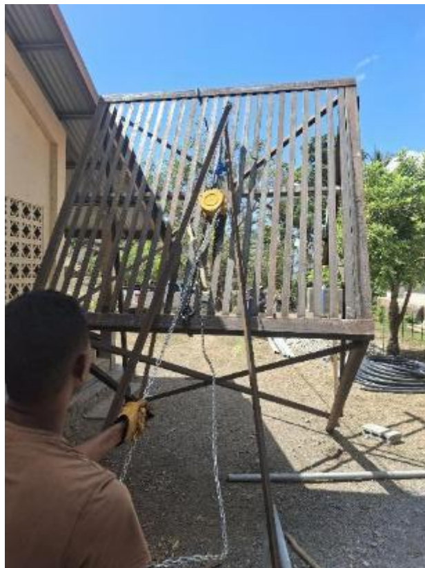
Using chain block and A-frame to safely lift tank stand into upright position
