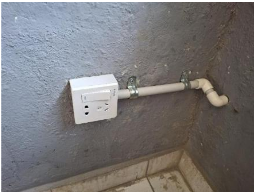
We added a mounting block and a new power point in a classroom., so we could hard-wire in our power supply to the pump.
