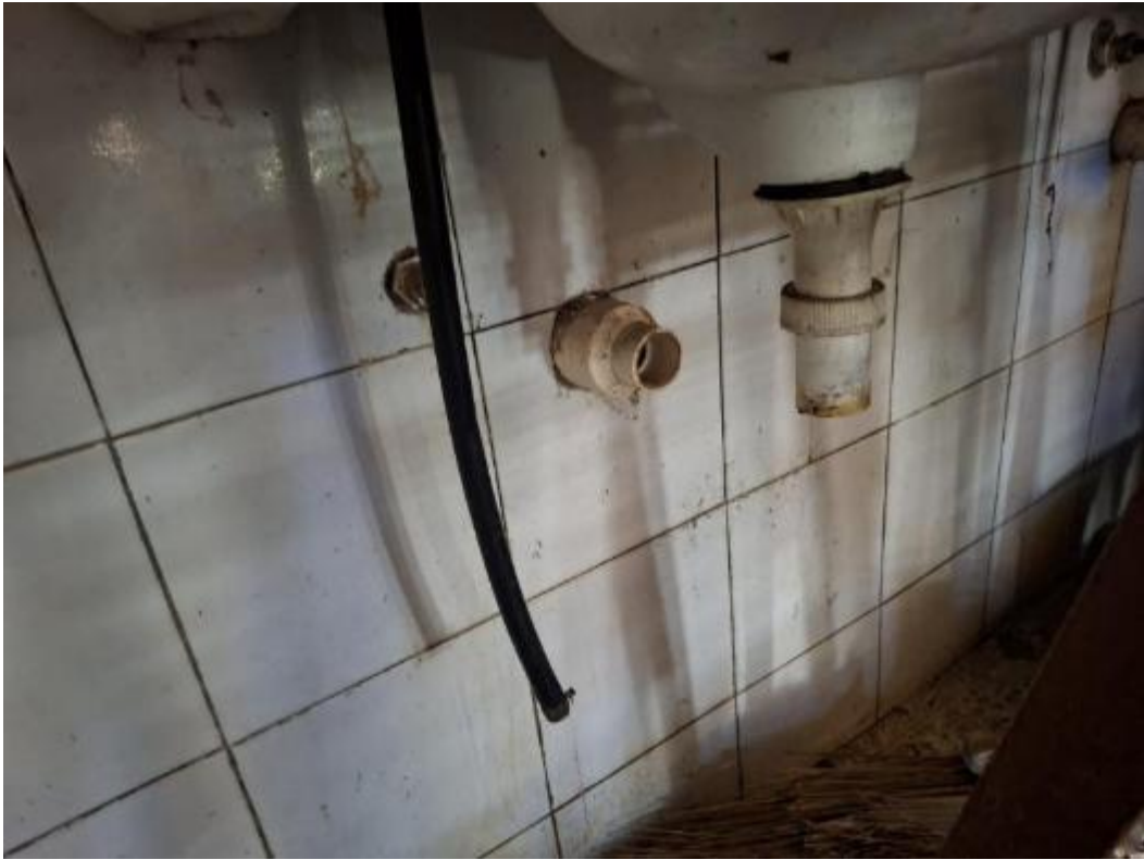
Same basins – no outlet drain and flexible inlet pipes broken
