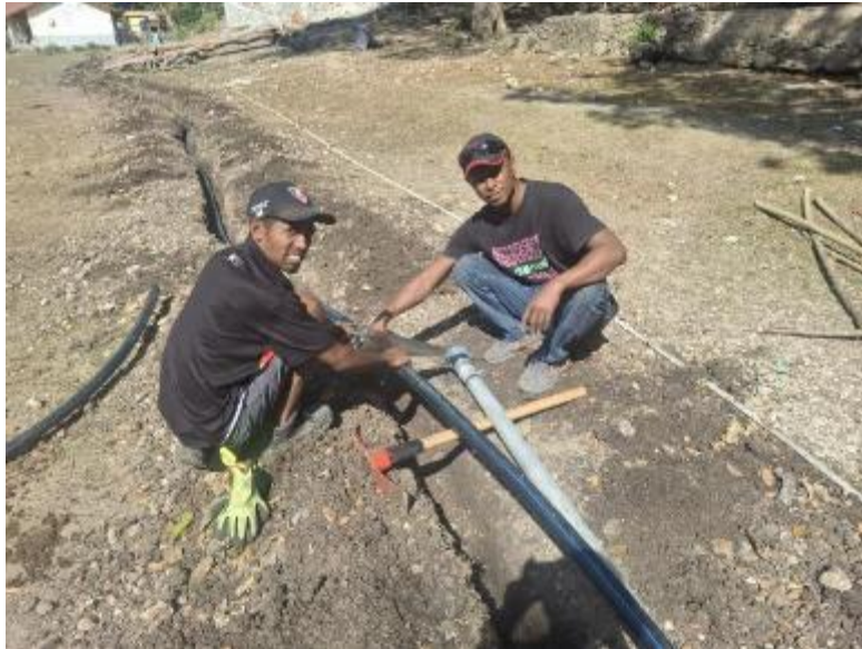
Mario (left) and San (right) attaching 50mm gal pipe to the poly pipe – with the gal pipe to go under the road.
