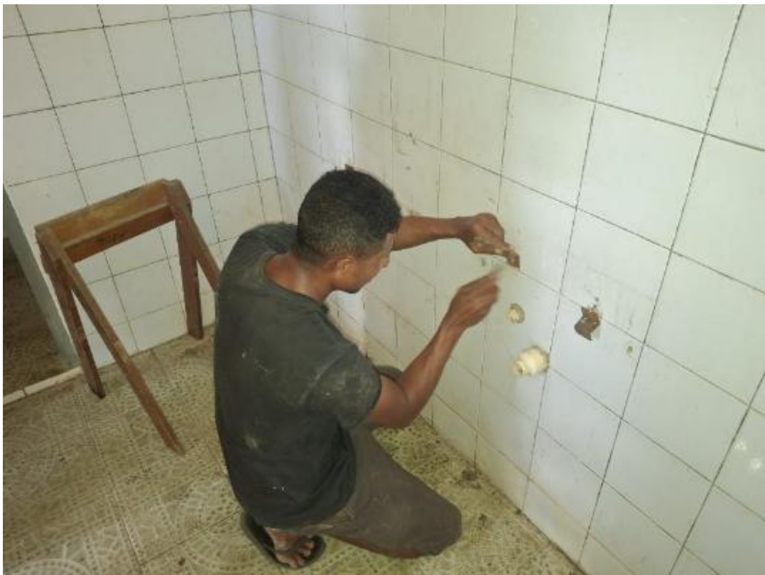
We removed the basins and San installed extra long screws in the brackets.
