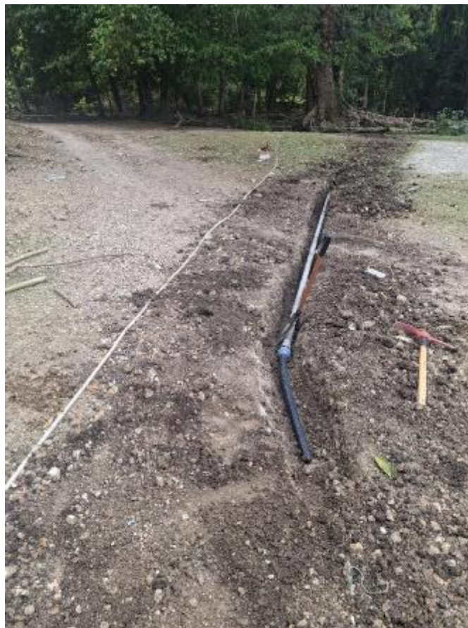
The gal pipe laid in the trench where the road passes over.
