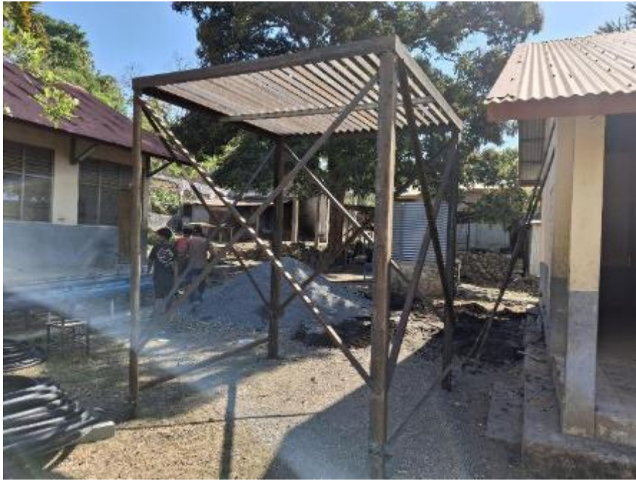
Tank stand ready to be moved into position into the pre-dug holes.
