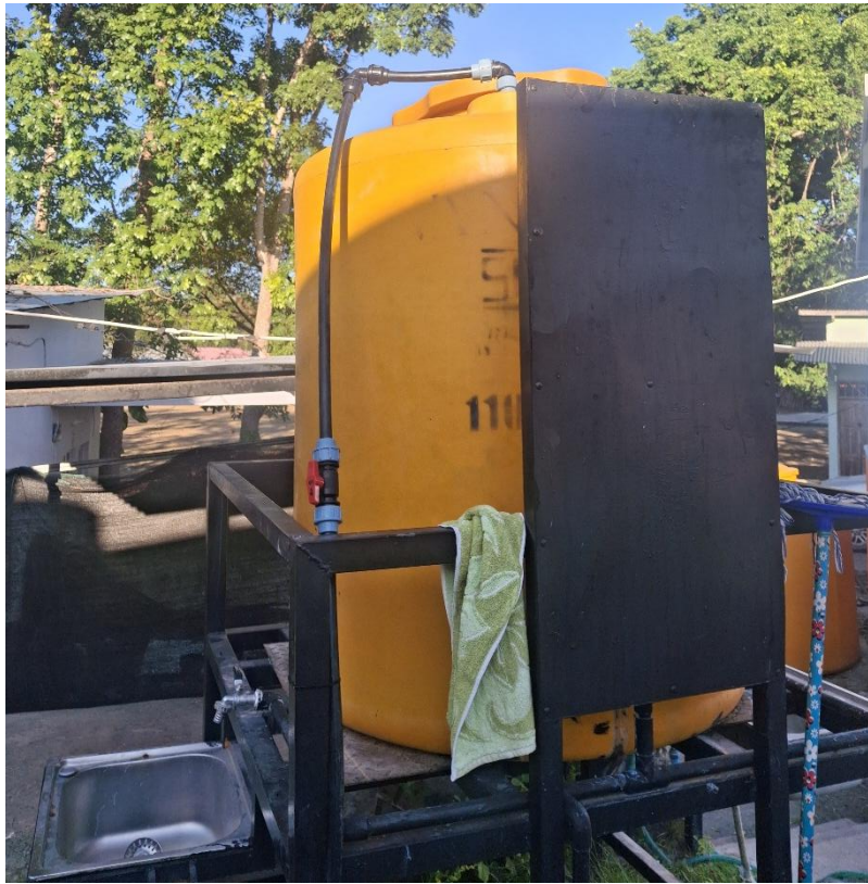
The Profile tank with supply line and tap, and new taps to the basins.
