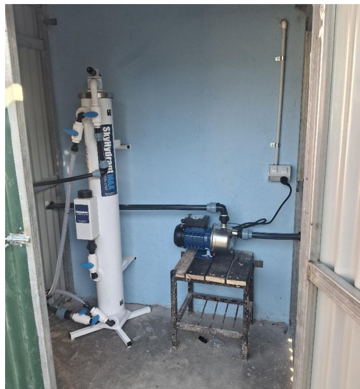
The SkyHydrant and pump in the shelter house.
