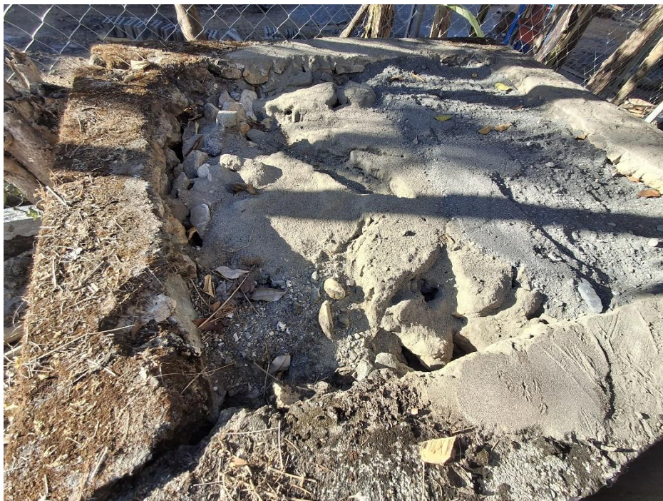
The base for the toilet tank. The space had been filled with large stones, but then sand laid on top, with no barrier between the two layers. Consequently, the sand then dropped down between the stones creating a very uneven base for the old tank.
