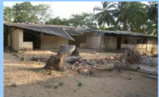
Orphanage Dormitory Buildings
