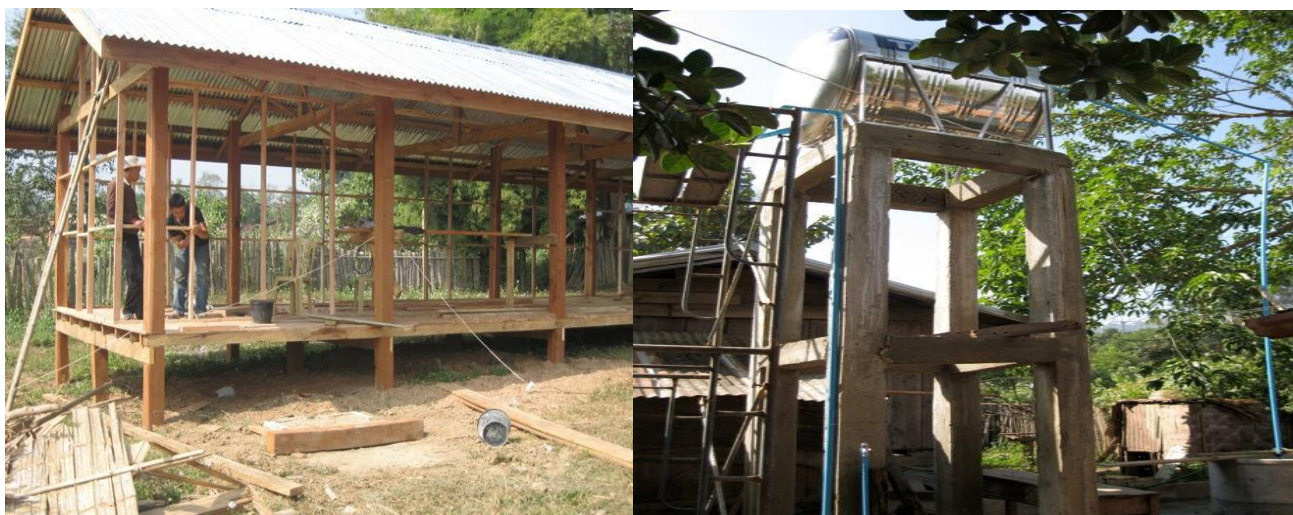
Accommodation Block under construction and Water Tower
